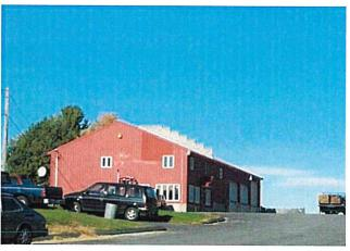
The next building, "B," to the left, is a red, metal-sided structure This corrugated steel building was built about 1987. It is divided into two sections by a concrete firewall. The half closest to the road was used as office space. To the rear is a maintenance area. It has an overall footprint of 40-ft x 100-ft (4.000 SF) of floor area and a total of 5,920 SF finished area, some on a second floor above the offices.
