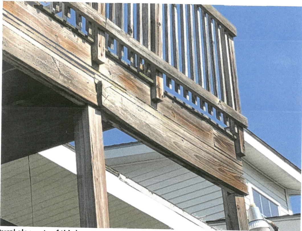
Structural elements of third story egress porch separating. Violation: Sec. 12-226. - Maintenance.
