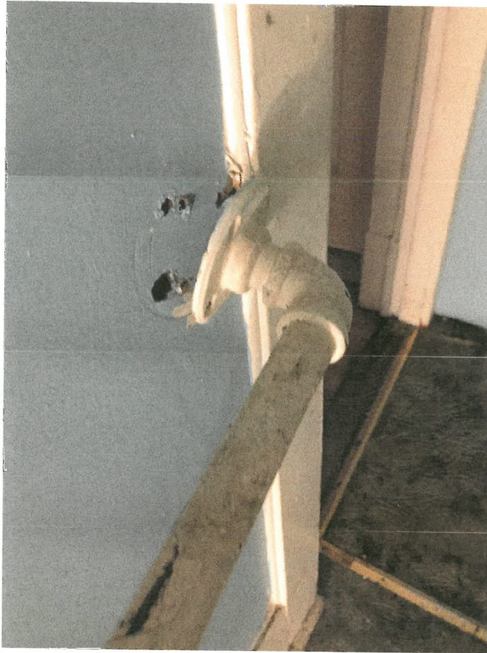
Broken loose handrail to second floor – Violation: Sec. 12-226. - Maintenance.
