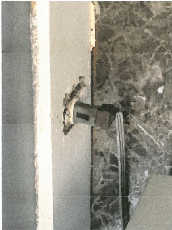
Unit #3 Electrical covers missing, and exposed wiring- Violation: Sec. 12-229. - Electrical and lighting.
