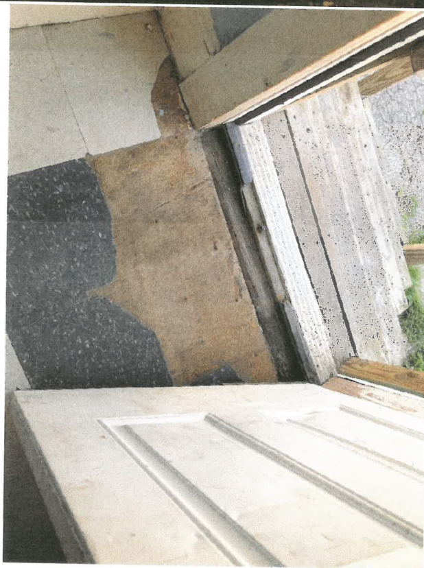
Common area to units #3 and #4 No floor covering or weather stripping around door Violation: Sec. 12-226. - Maintenance.
