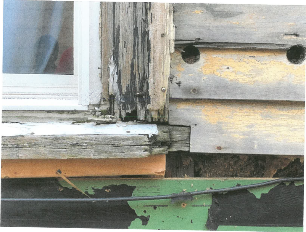
Rotten windowsill above where new beam was installed below. Violation: Sec. 12-226. - Maintenance.
