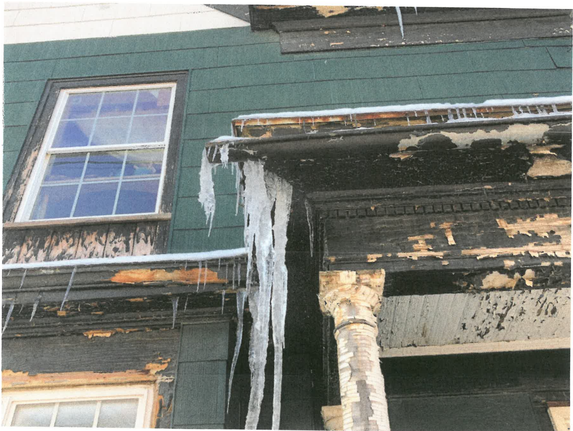
Violation: Chipping and peeling paint and water damage Sec. 12-226. - Maintenance.
