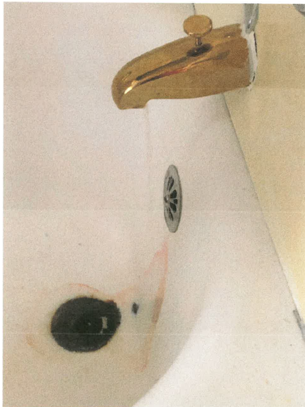
Unit #3 Leaking plumbing/faucet- Violation: Sec. 12-227. - Plumbing.
