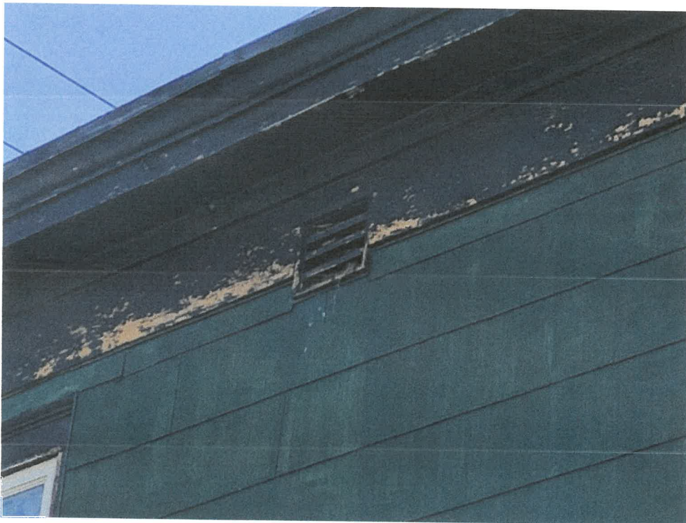
Attic vent blocked with nest/rodents - Violation: Sec. 12-228. - Heating and ventilation.
