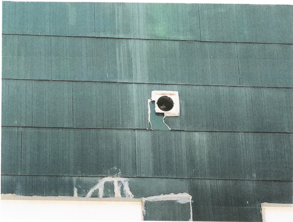
Broken dryer vent- Violation: Sec. 12-228. - Heating and ventilation.
