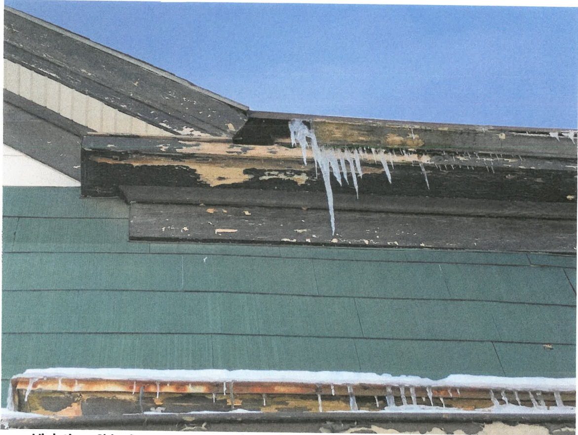
Violation: Chipping and peeling paint and water damage Sec. 12-226. - Maintenance.
