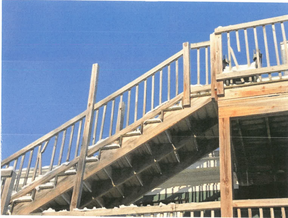
Violation: Exterior rear egress stairs with broken guards structural members separating Violation Sec. 12-226. - Maintenance.
