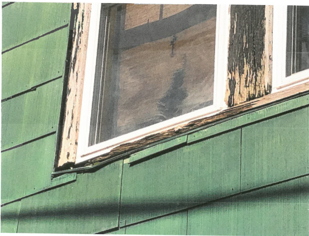
Missing trim/facia allowing water intrusion on structural elements- Violation: Sec. 12-226. - Maintenance.
