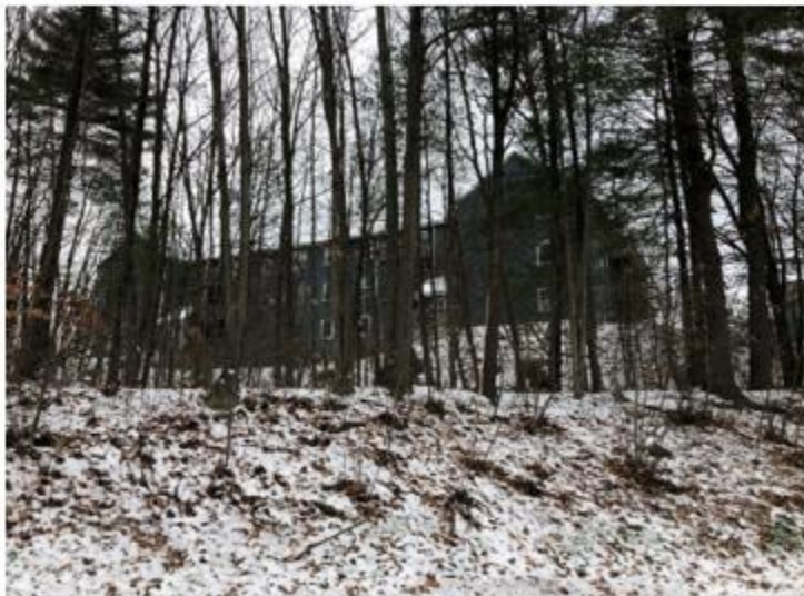
View of Northern Avenue Heights Development from N. River Road
