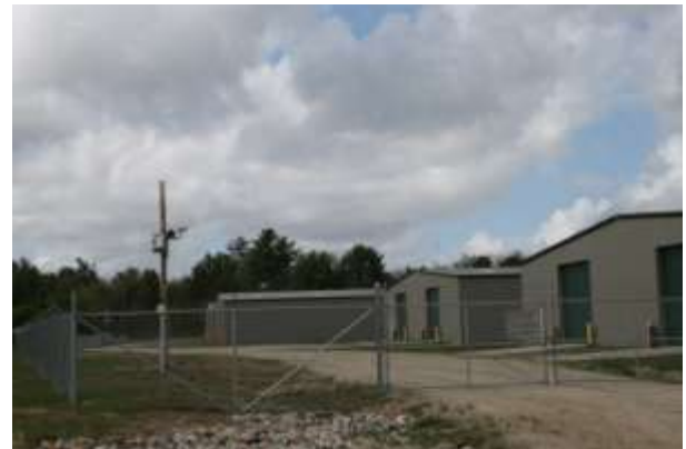
Figure 1.5 Controlled humidity preservation buildings
