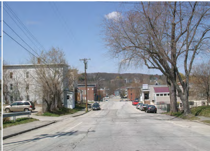
Second at Dunn looking towards Auburn
