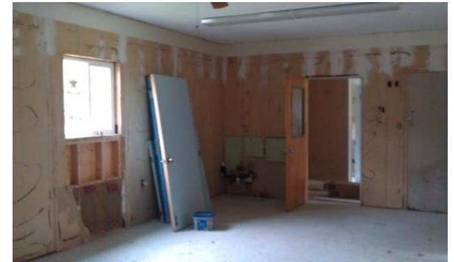
Interior of PAL Center awaiting renovations
