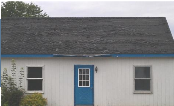
Auburn PAL Center before renovations
