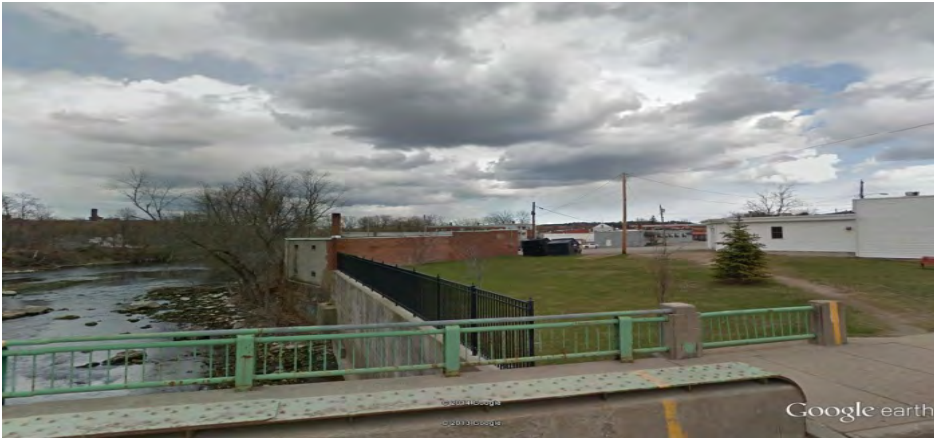
South Main Street, downstream side of Main Street bridge over the Little Androscoggin – Replaced a stone wall and was constructed in 1996.
