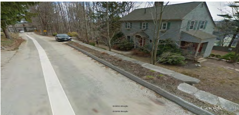
72 Hillcrest Street – Stone wall constructed in 1994.
