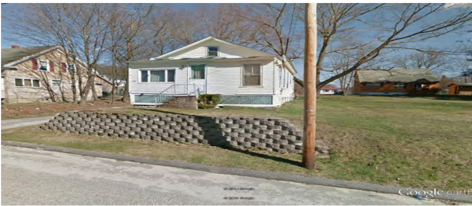
42 Taft Avenue – Keystone Block wall constructed in 1995.
