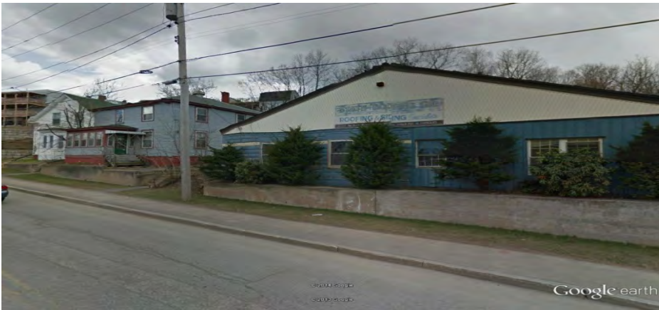
21 to 33 South Main Street – Concrete wall constructed in 1955.
