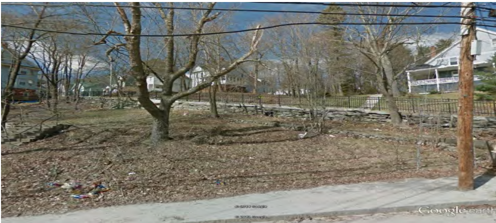
18 Western Prom – Stone wall constructed in 1887. The City added a fence to the top of the wall in 2013.
