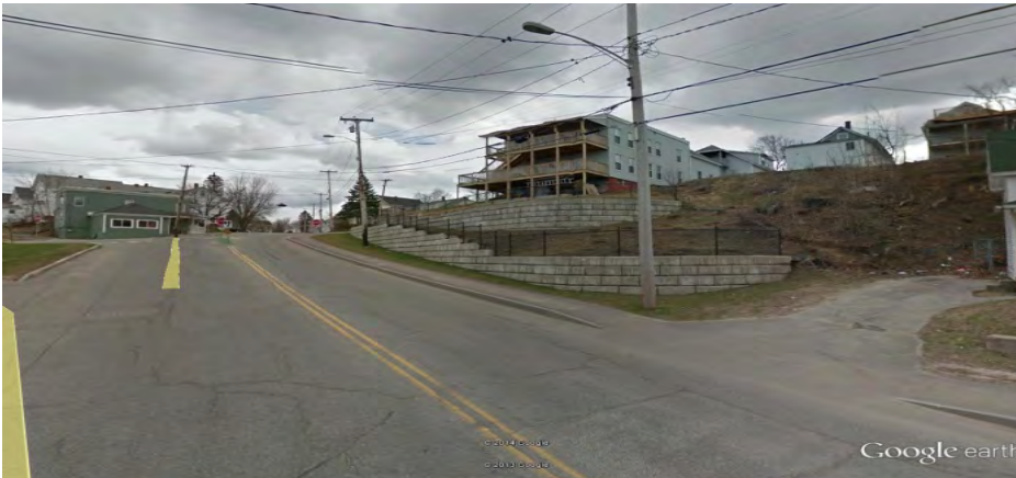
South Main Street, Broad Street Intersection – Redi-rock wall constructed in 2008.
