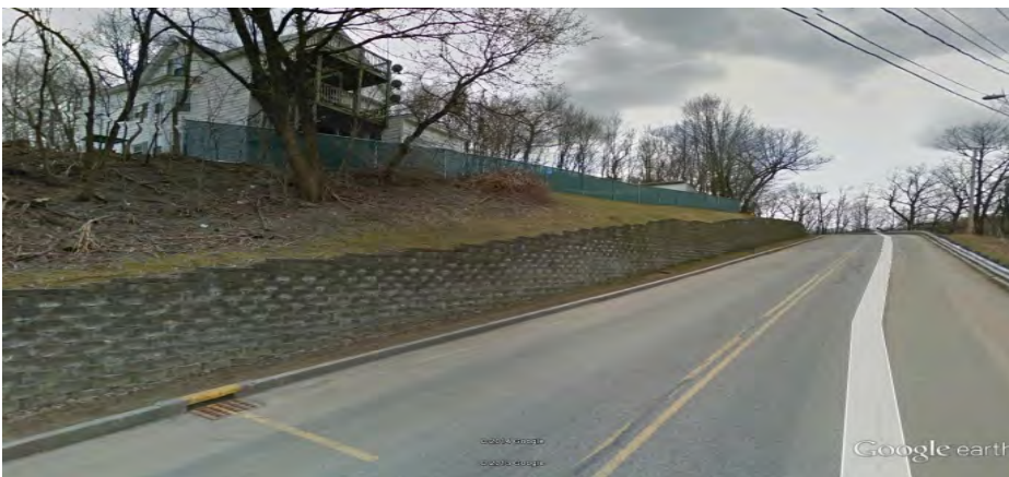
Mill Street, Sixth to Seventh – Keystone Block wall constructed in 1998.
