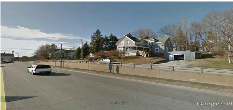
Washington Avenue, between Minot Ave. and Jefferston St. – Concrete wall constructed in 1957.
