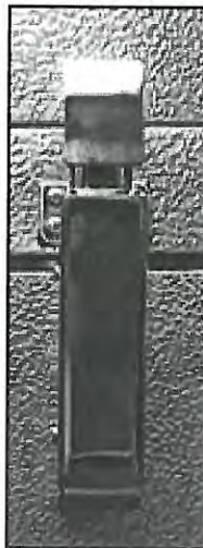
SPRING ACTUATED DOOR CLOSER
