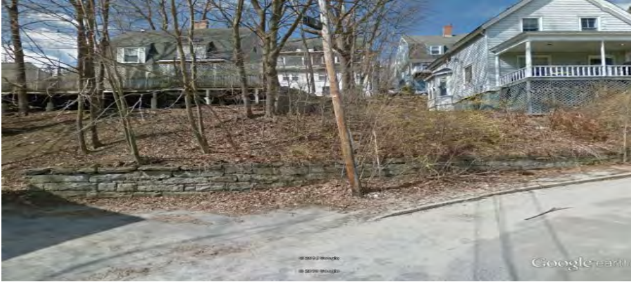
Charles Street, West side – Stone wall construction date unknown.
